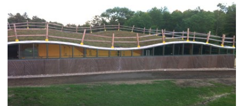
Shortly after completion: The "Biomass Treatment Center" with its green roof.
