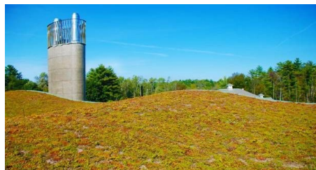
Due to the use of precultivated sedum mats, the roof was covered by vegetation quickly.
